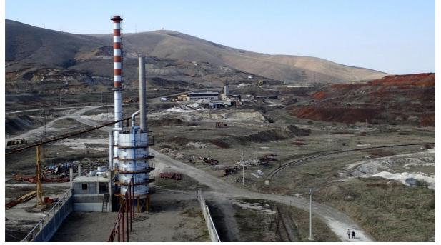
Figure 12-20 Vertical kiln, in the back the shaft (gallery) and processing plant
