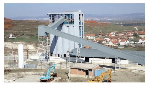
Figure 12-13 MgO product silos with belt from rotary kiln to silos
