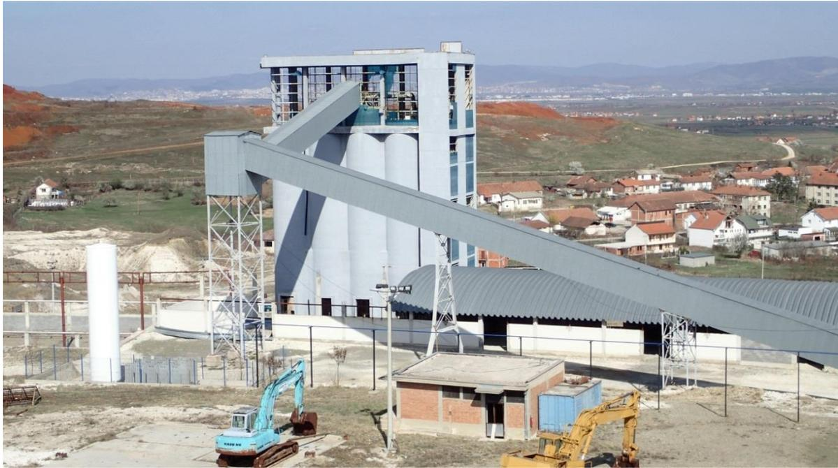
**Figure 12-13 MgO product silos with belt from rotary kiln to silos**
