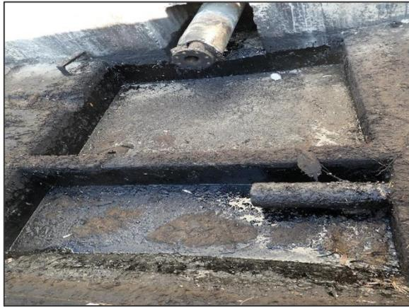
Figure 13-3 Oil separator at fuel storage area
