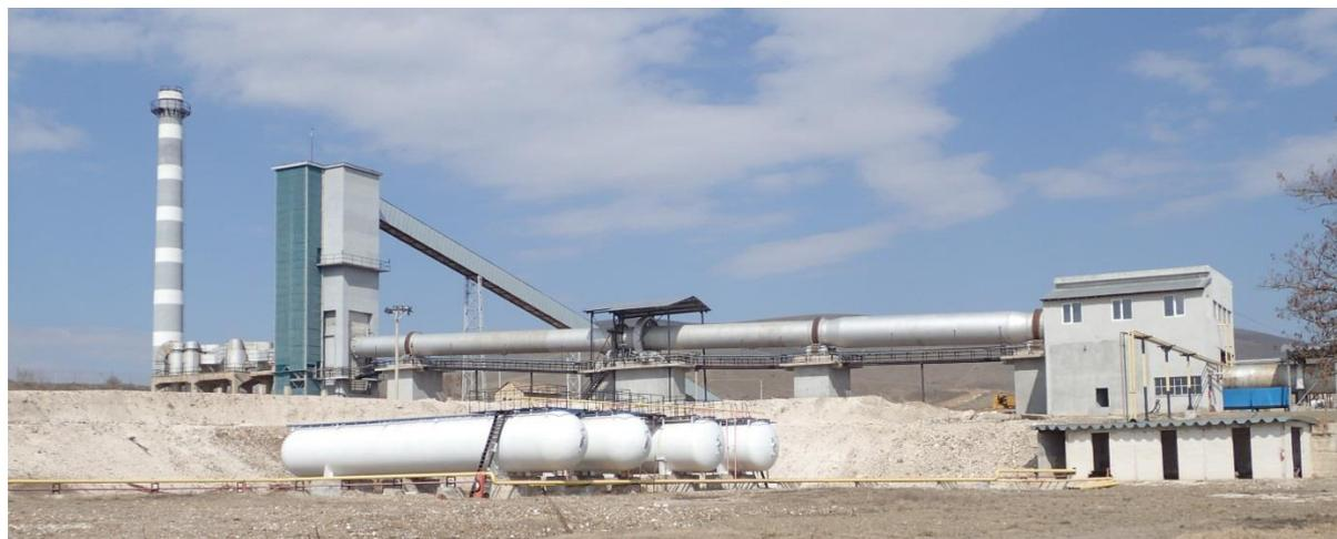
**Figure 12-15 Rotary kiln during site visit in March 2019, in front the new gas tanks (Propane 70% and Butane 30%)**
